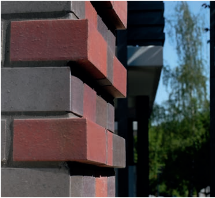
Building corner with ledge, Buchsbaumweg, Hamburg
